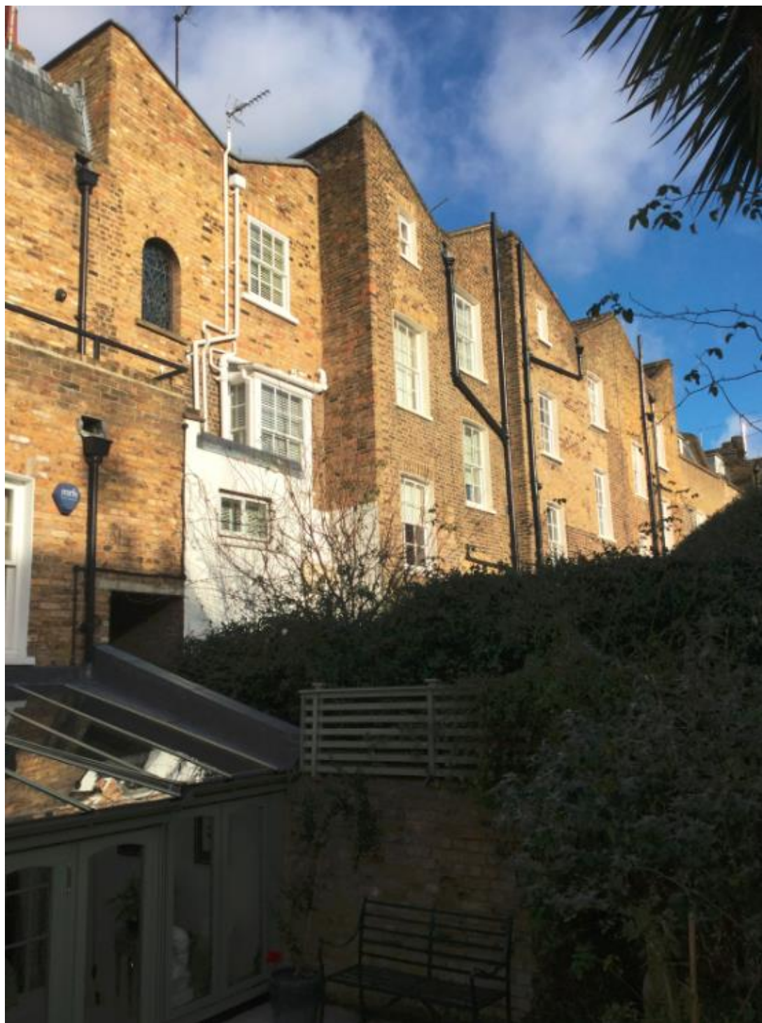
Rear of Application Property. The objector's property at No.14 is to the left.
