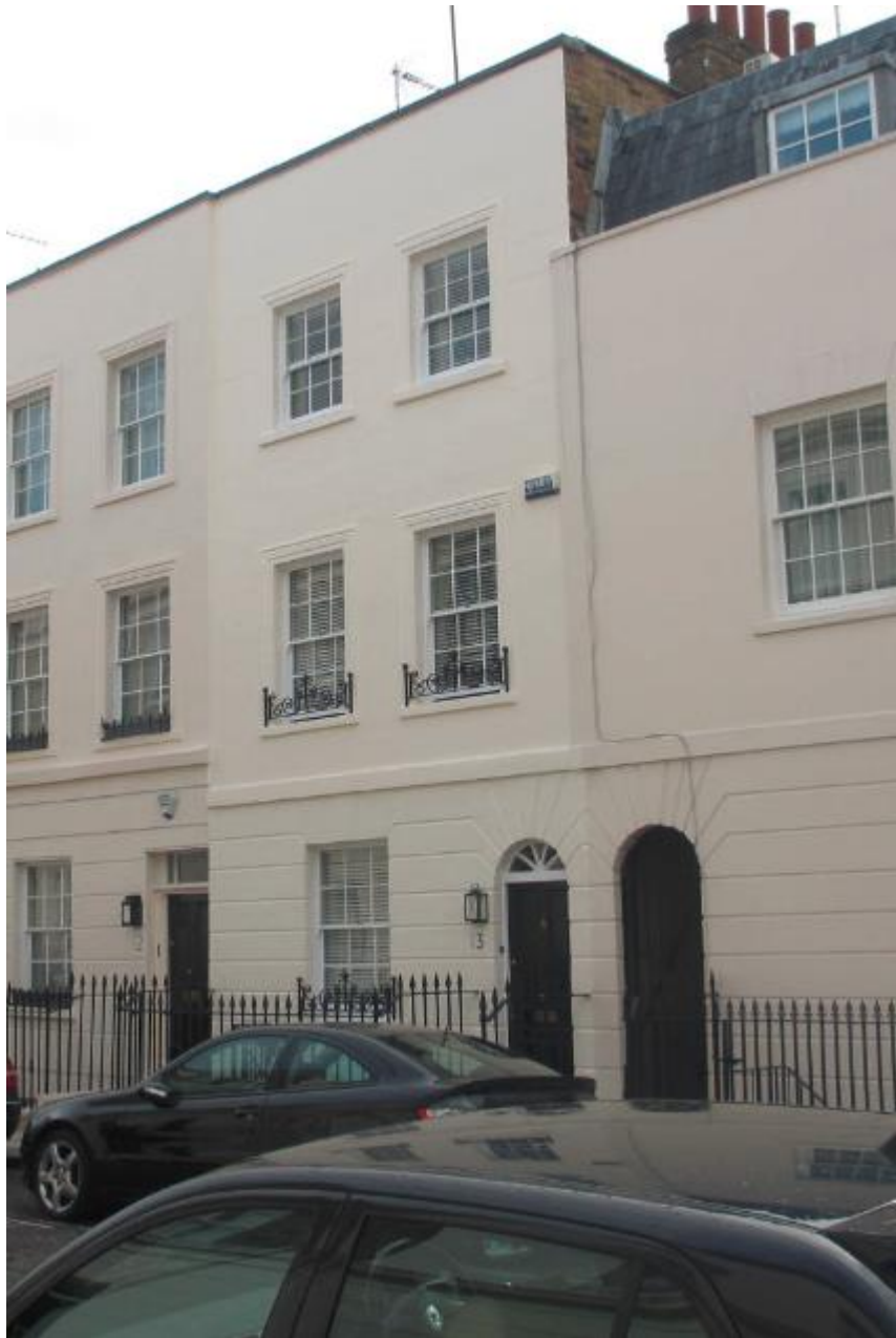
Front of Application Property
